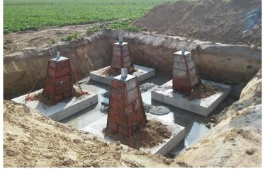
Fig. 2. Monolithic foundations intended for a 72-meter-high power pole of a 400 kV line (*own photo*)
