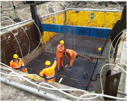
Fig. 5. Installation of foundation reinforcement (own photo)
