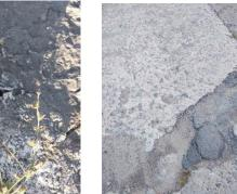
Fig. 2. Destruction of joints between reinforced concrete slabs
