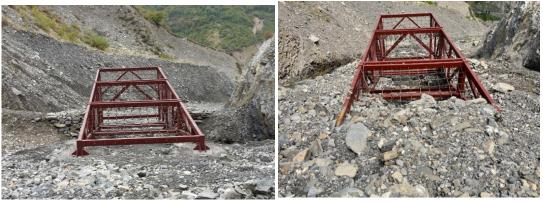
View of the structure before the debris View of the structure after the debris flow flow passage passage Fig. 9. General view of the debris flow regulation elastic barrage regulating solid fractions
