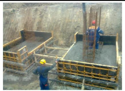
Fig. 7. Filling the foundation "chimneys" with concrete mixture. The visible anchors on the gables are connections to the structure (*own photo*)
