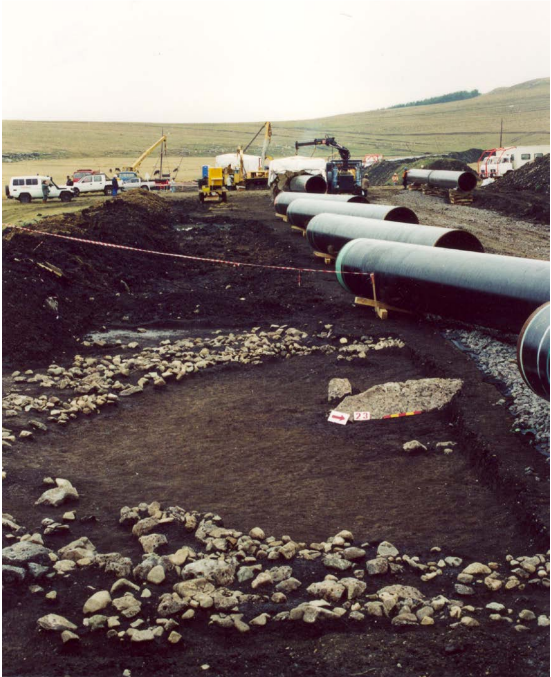
Pic. 27. Construction activities on KP-120
