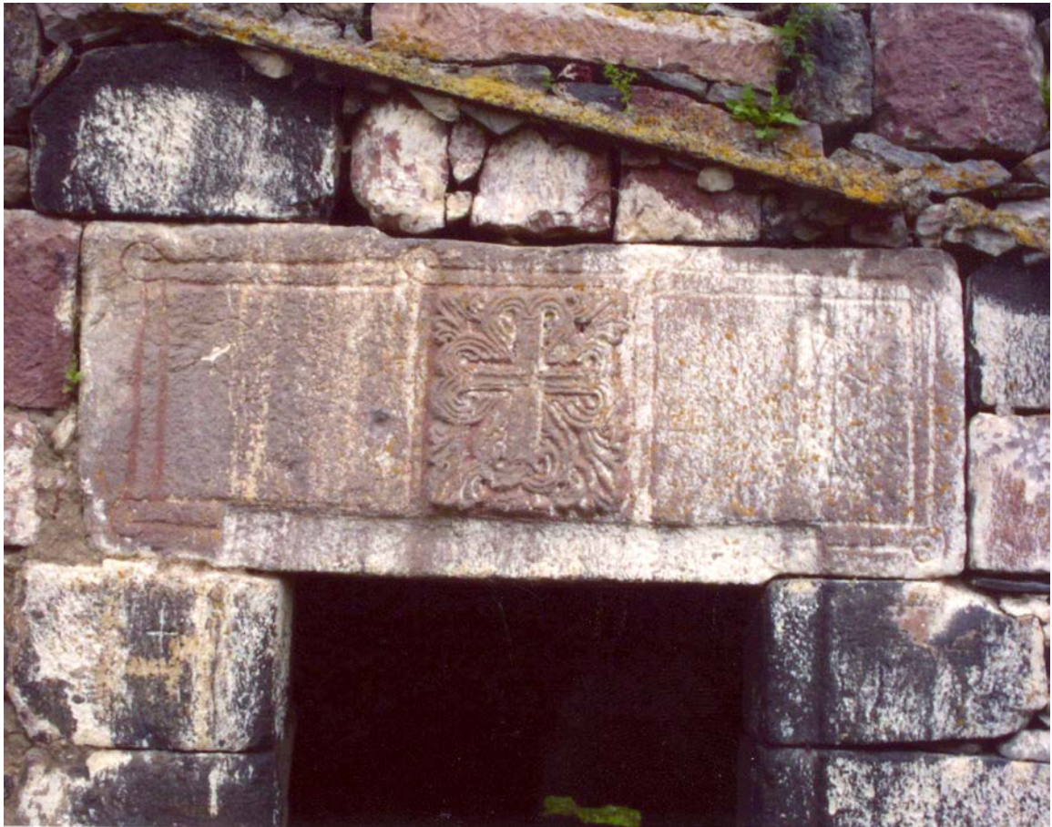
Pic. 339. Sapitiakhsho. Entrance. Detail.
