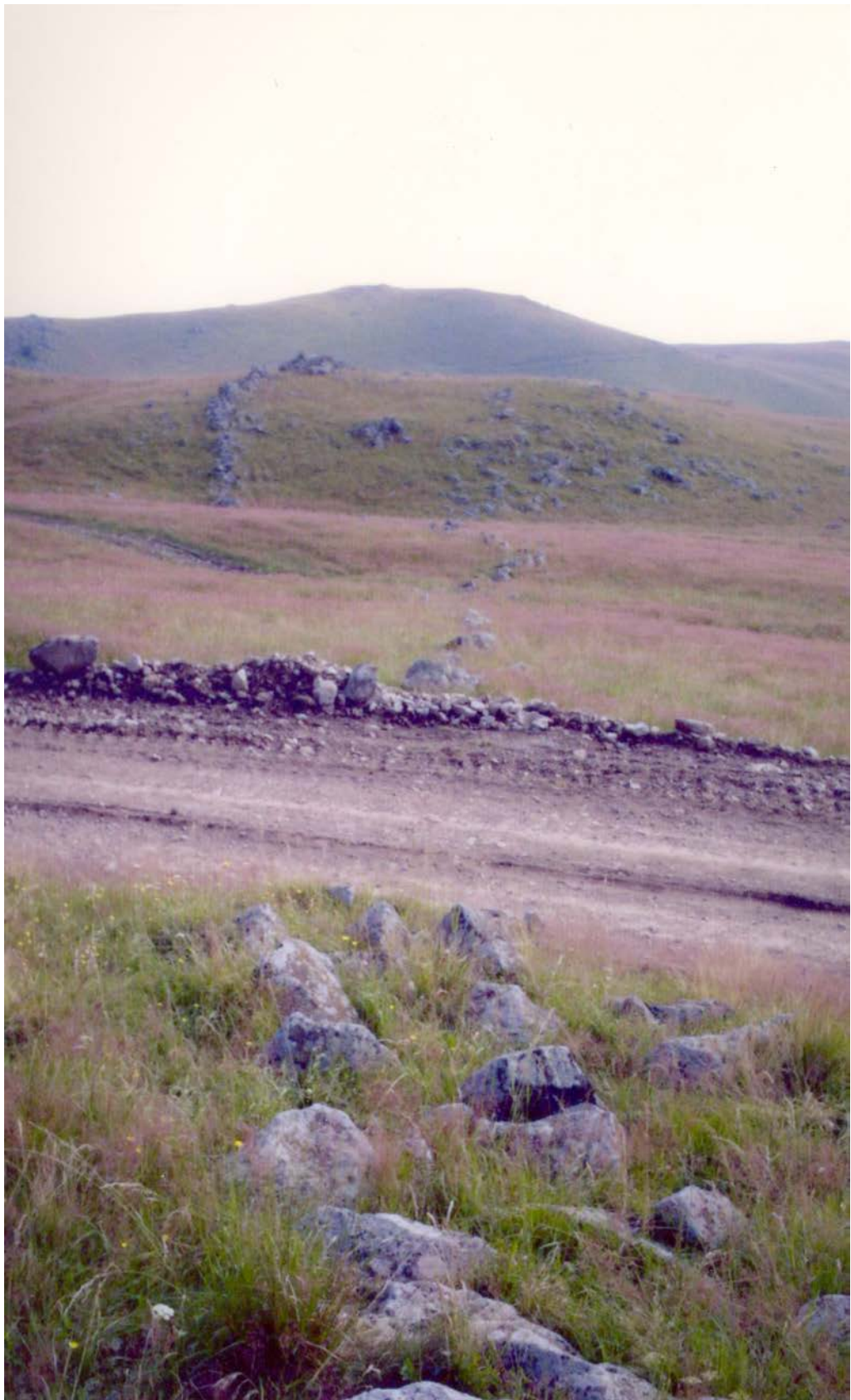
Pic. 351. Sapitiakhsho. Wall. General view
