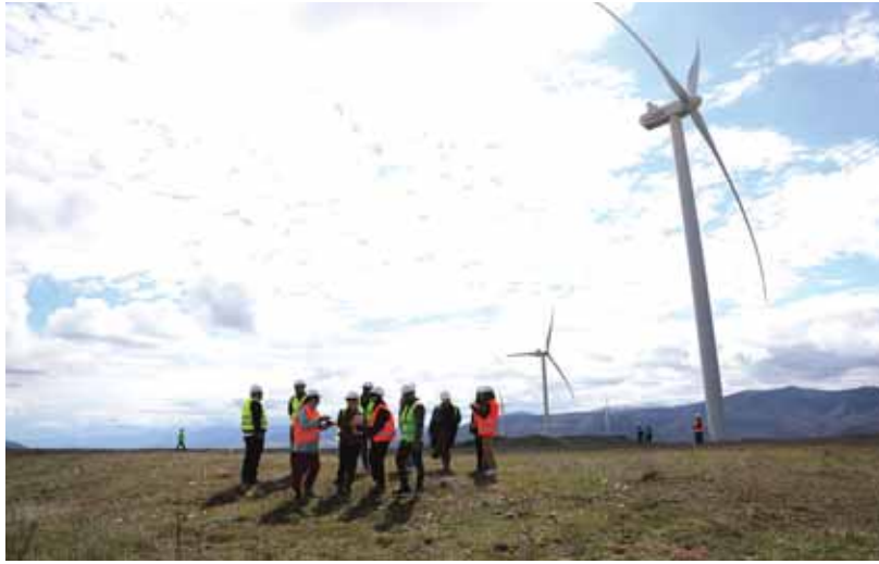
The Gori wind plant
