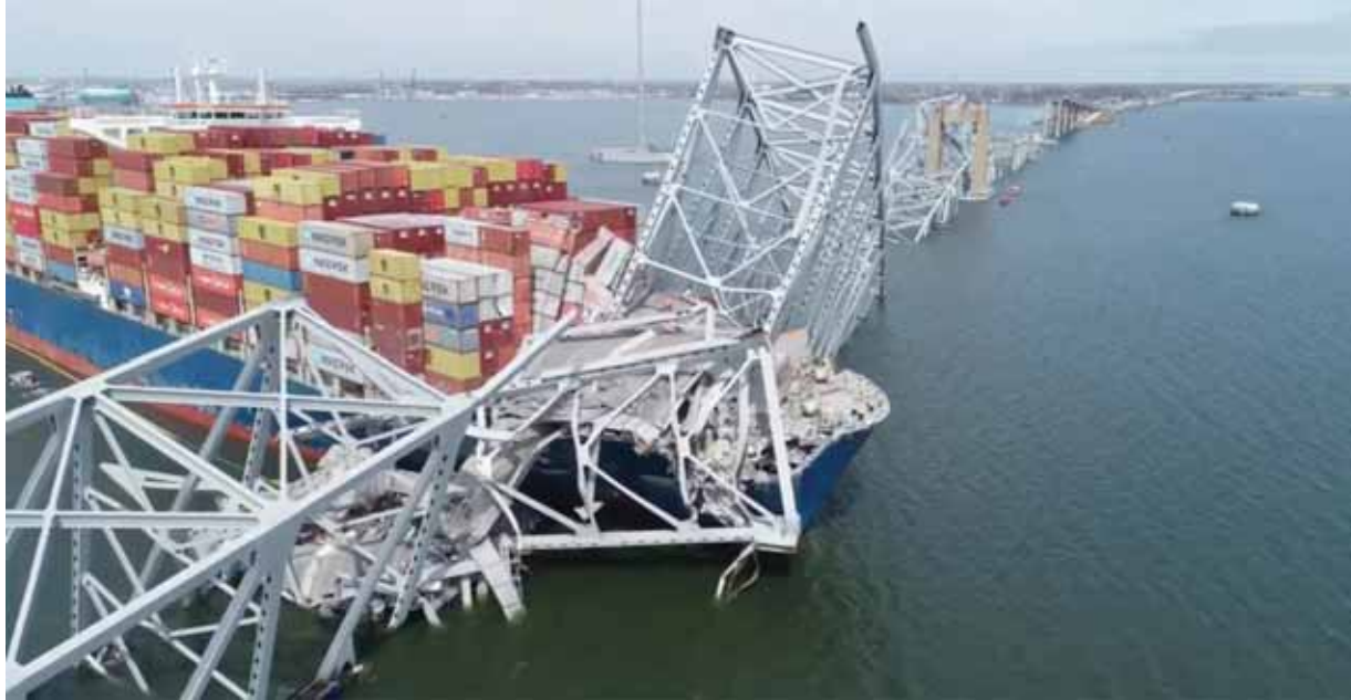
The Singapore-flagged container vessel named Dali, heading out of Baltimore Harbor bound for Sri Lanka, lost power and plowed into the Francis Scott Key Bridge at about 1.30am on Tuesday. Six workers were killed. Source: REUTERS
