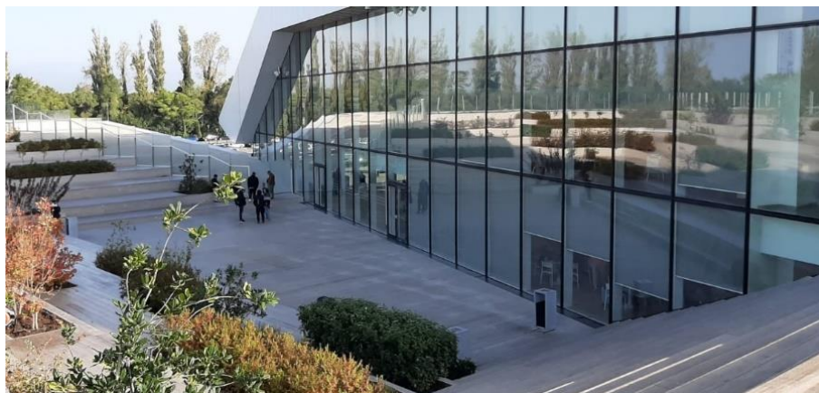
Fig. 3. Green roof of the Kutaisi airport building [Photos: Kutaisi International Airport and taken by the authors]
