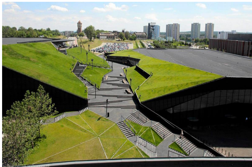
Fig. 9. Green roof over the International Congress Centre in Katowice [22]
