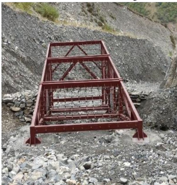
View of the structure before the debris flow passage
