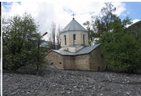
Fig. 4. Yard of the Church of Mleta covered with debris flow mass and solid fractions
