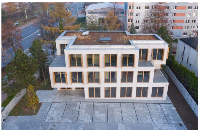
Fig. 12. Green roof over the EXG office building in Częstochowa [25]
