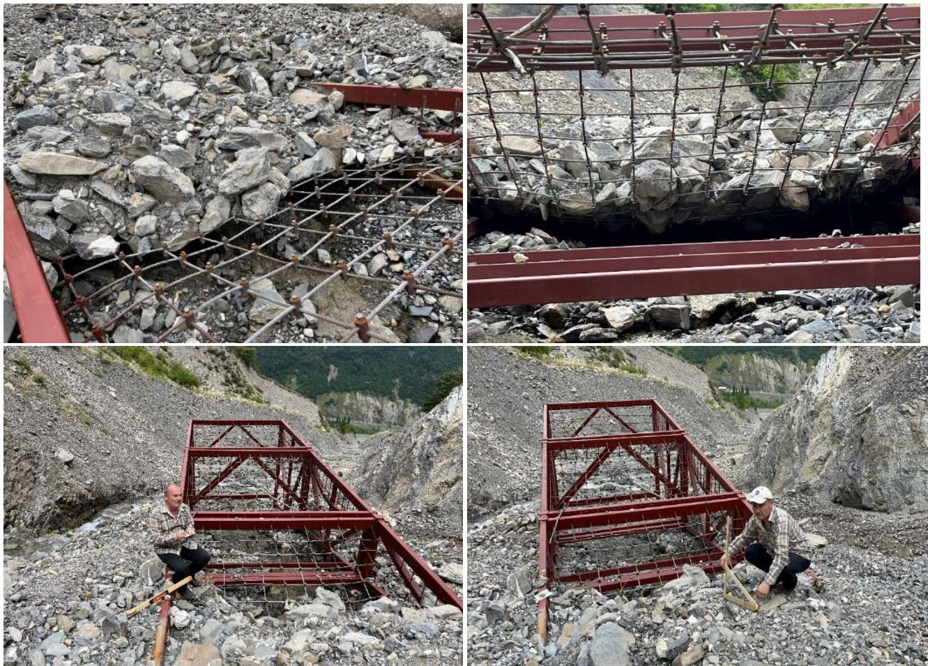
Fig. 13. General view of the debris flow regulation elastic barrage
