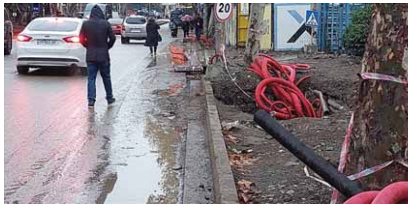
Tsereteli Avenue, works in progress. Photo by Aleksandre Devadze
