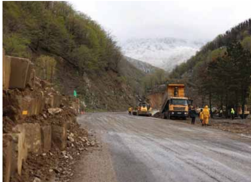
The Rikoti Pass. Source: Facebook, Georgian Roads Department
