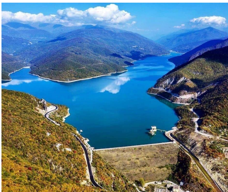
Fig. 1. General view of the Zhinvali reservoir
