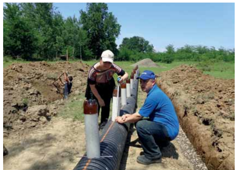
During the construction of three-tiered combined drainage
