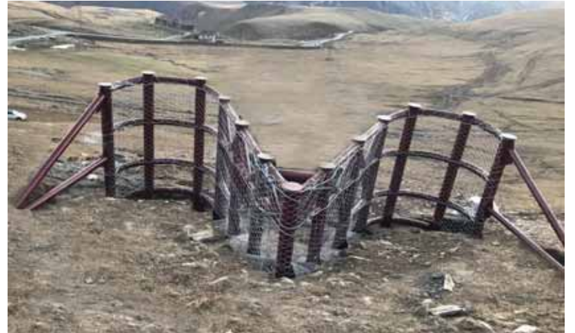
Innovative construction anti-snow avalanches (2021)
