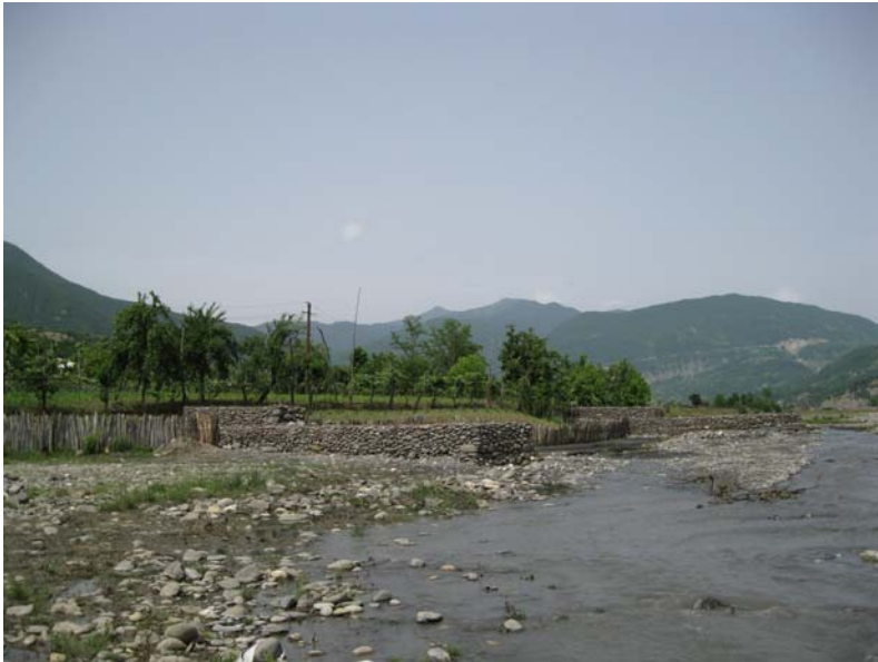
Fig. 11. Stone anti-flood spurs on the Tskhenistsqali river. Tsageri. 23 May 2009.
