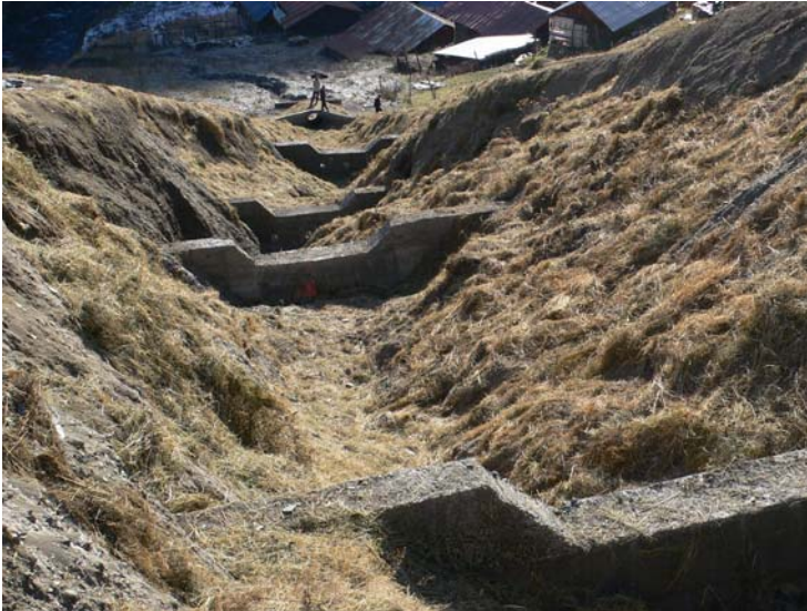
Fig. 7. Concrete antierosional barrages. Mountainous Tusheti. 21 November, 2007.
