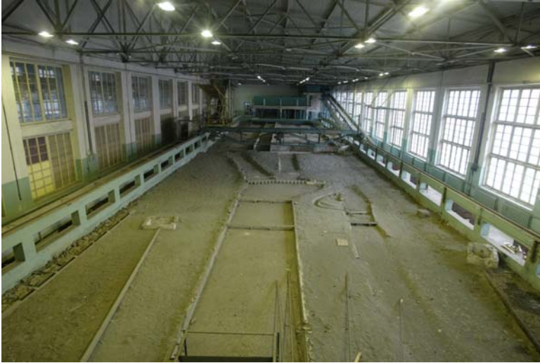
Fig. 1. The hydrotechnical laboratory
