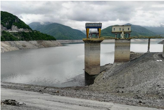
Fig. 2.5. Head-water of Zhinvali earth dam with water intake structure
