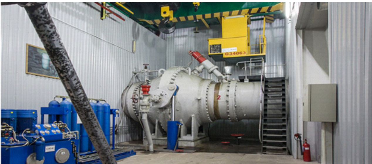
Spherical lock building
