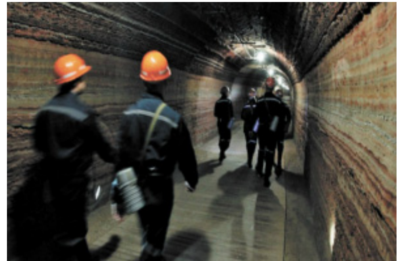
At the decision of the Labour Inspection Service of Georgia, the site where the explosion took place will close down.
