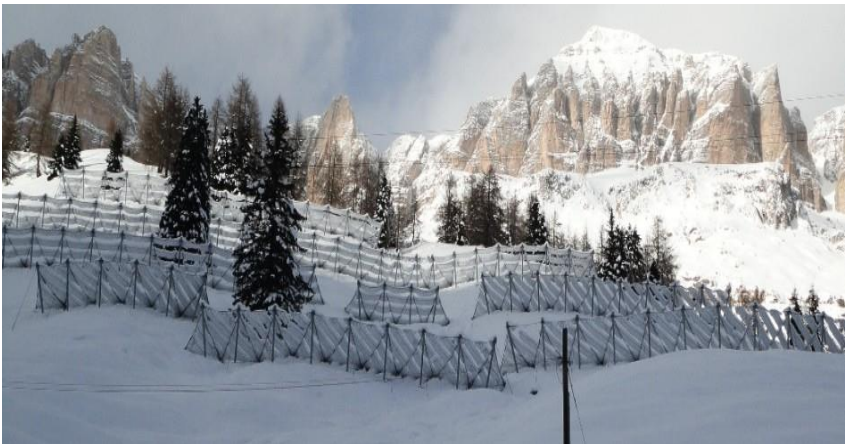
Photo 2.1. Flexible CTR-OM snow barrier rows in the Alps
