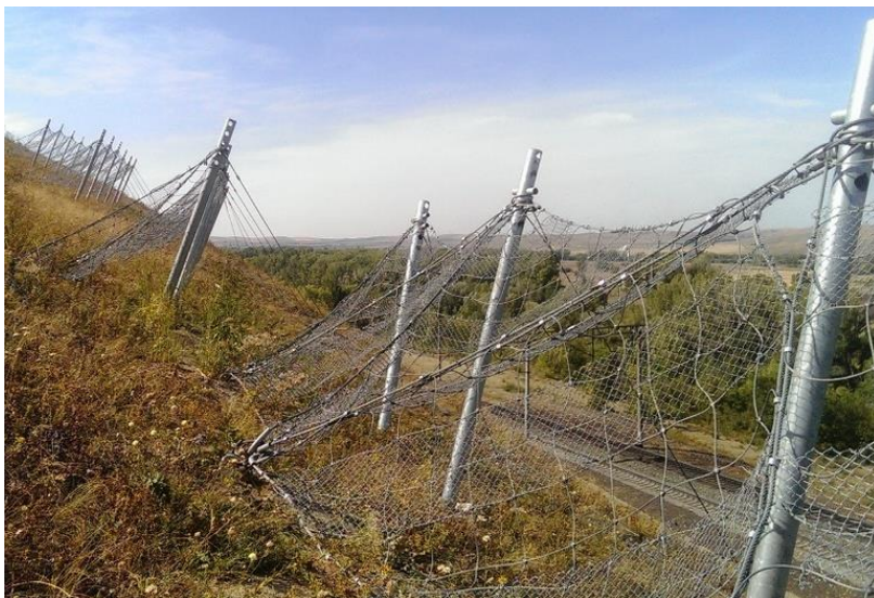
Photo 2.2. CTR-OM system anti-snow avalanche barrier
