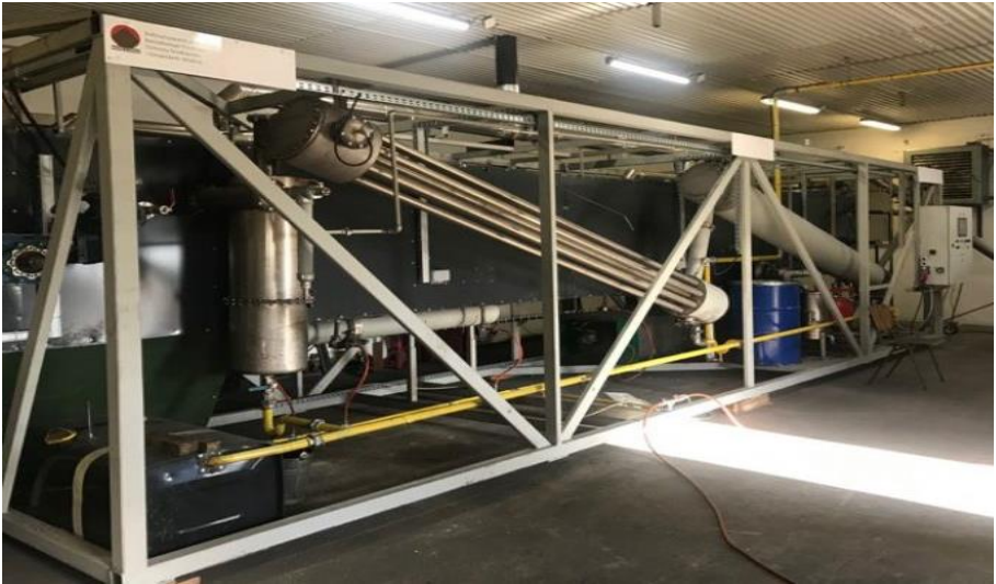
Fig. 1. Installation of waste pyrolytic transformation
