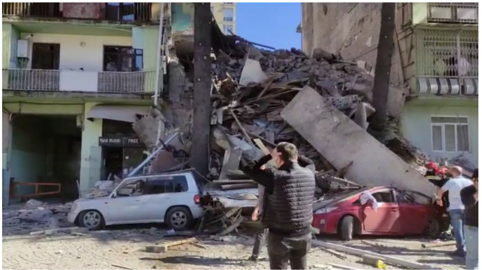
The building on 26 May street collapsed on October 8
