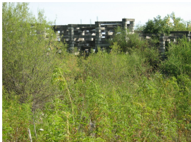
Fig. 7. Mudflow-holding through construction
