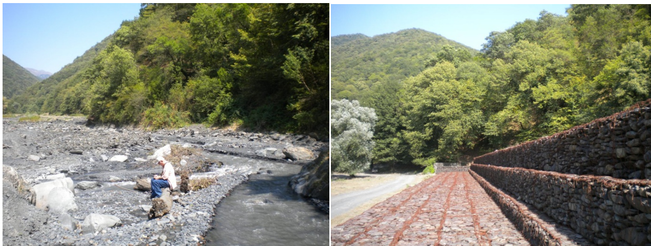
Fig. 5-6. The Duruji River mudflow material leaving the canyon area and a bank-protection gabion
