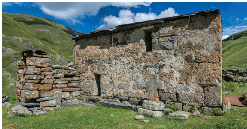
Mna Church of the Virgin, Southern façade
