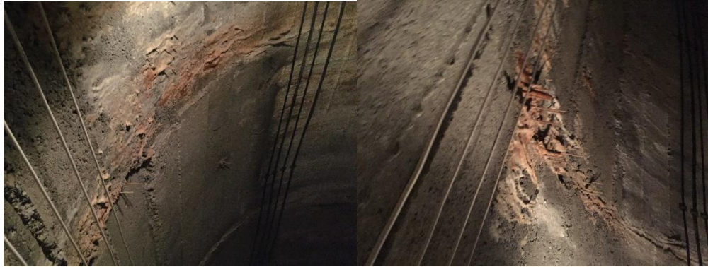
Fig. 3. The emergency sections of underground tunnel
