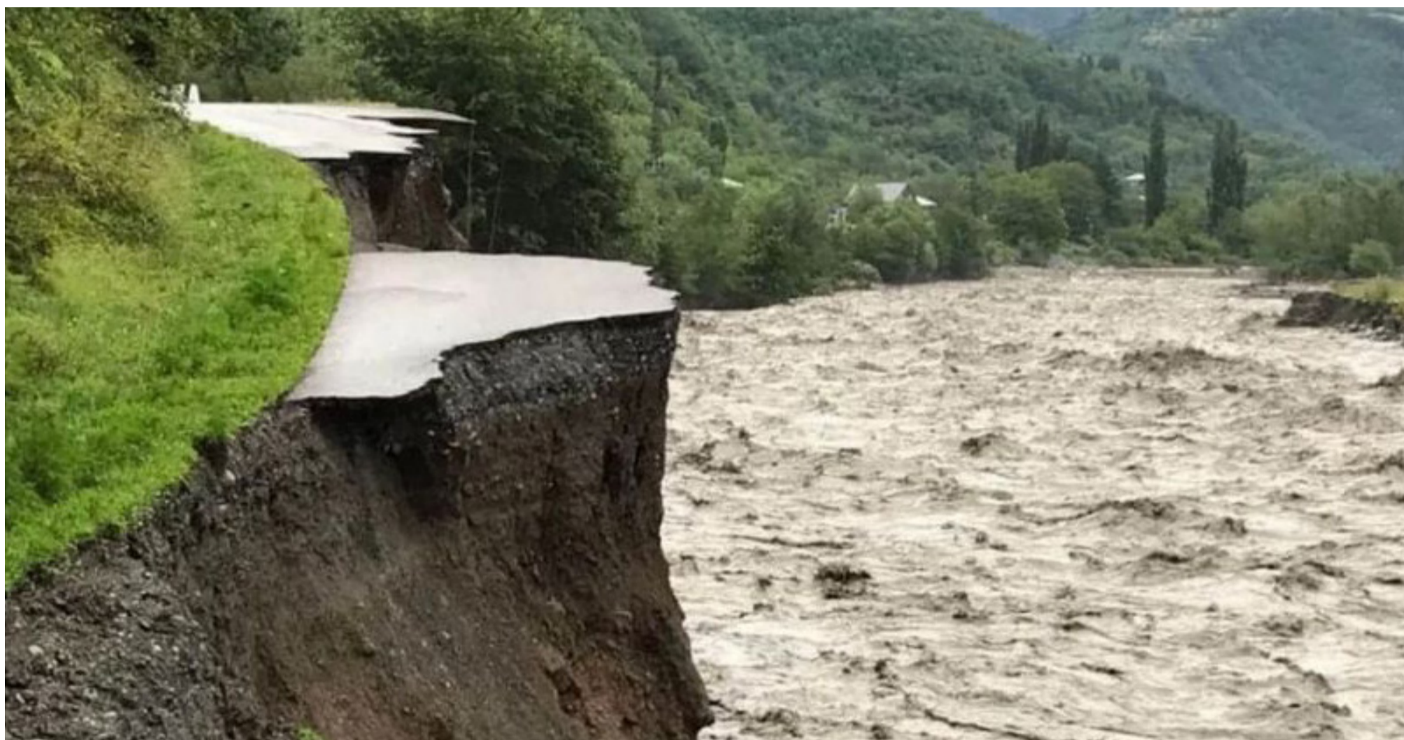
► Overflowing River in the Municipality of Oni
