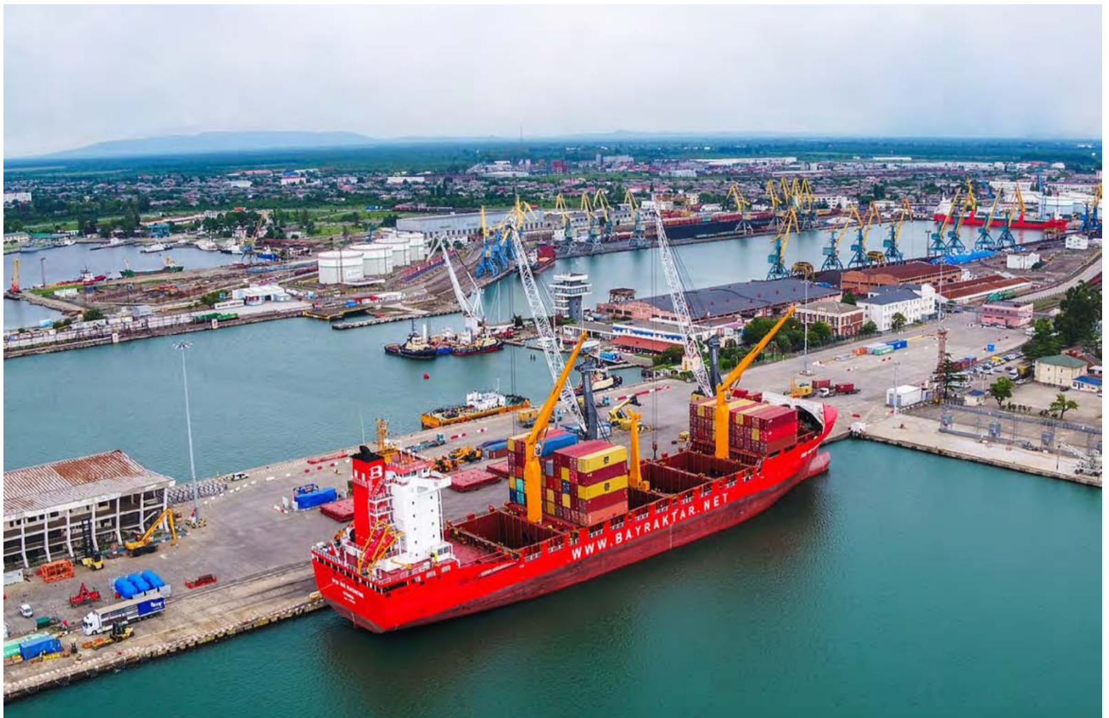
► The increase in construction was mainly due to infrastructure projects (roads, highways, bridges), which are mainly funded by the state. Photo: AP Terminals
