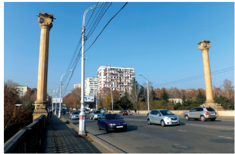
Didube bridge in Tbilisi
