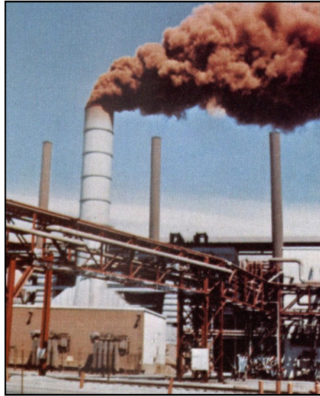
Figure 8. Red clouds of nano ferric oxide produced when oxygen was introduced in converter.
