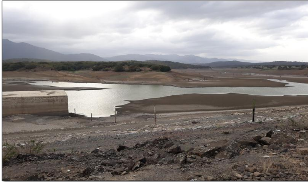
Fig. 1. Vilashchay water reservoir
