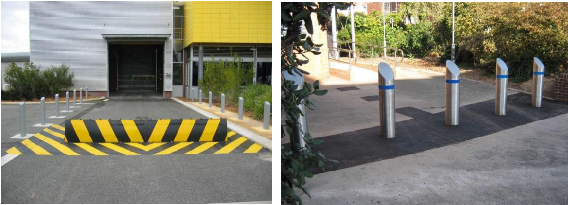
Figure 2 - Anti-RAM Barriers to prevent penetration of vehicles
