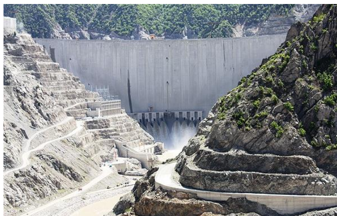
Fig. 2. Derineri Arch Dam on the Chorokhi River (Turkey)
