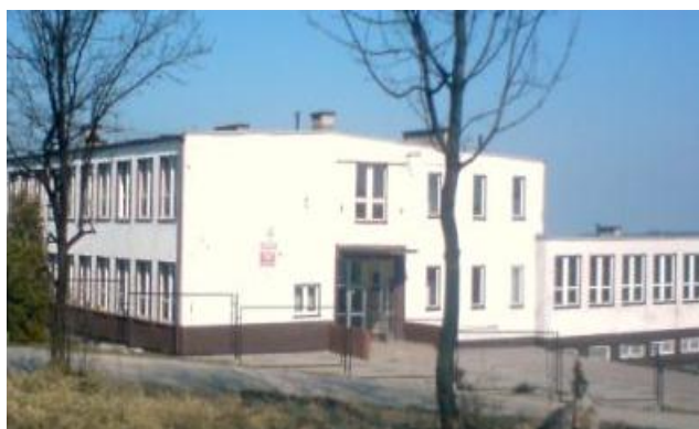
Figure 5. The school building before thermal modernization in 2006
