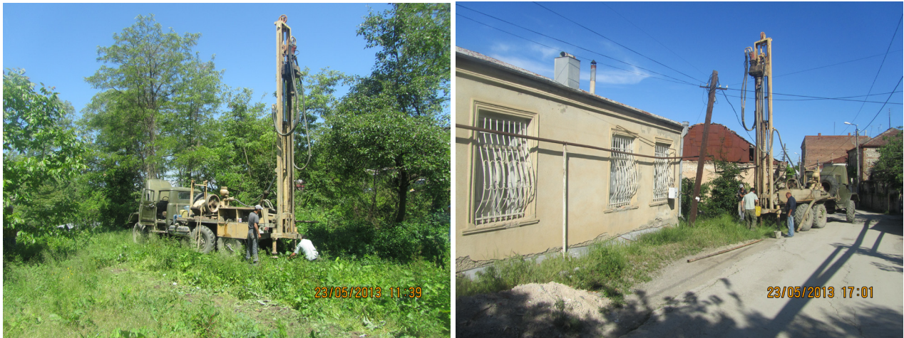
Fig. 3. Drilling the first and third boreholes
