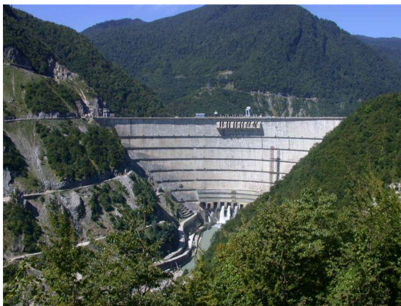
Fig. 2. General view of the Inguri arch dam
