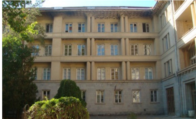
The highest category sanatorium named after Lazarev in “Arzni” resort, centralized scheme, Architect Samvel Safaryan
