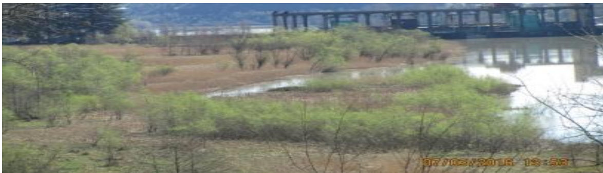
Pic. 2.4. The view in front of Gumati reservoir power intake
