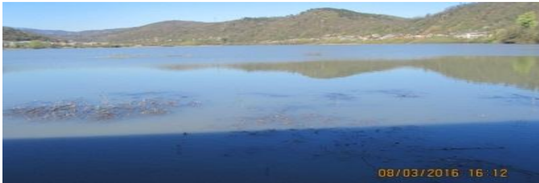
Pic. 2.5. The silted area of the Rioni HPP dam reservoir
