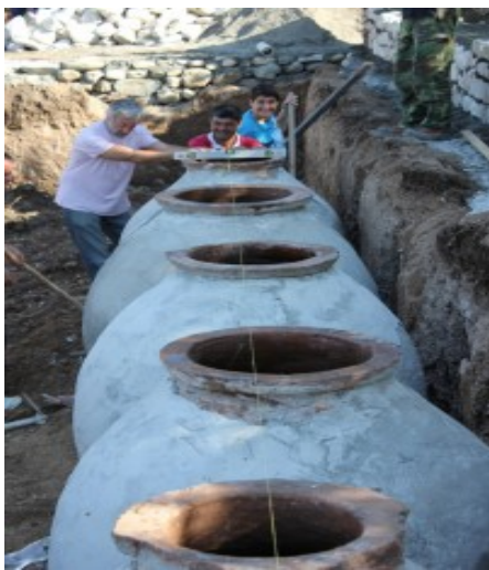
Installing Quevri at the winery
