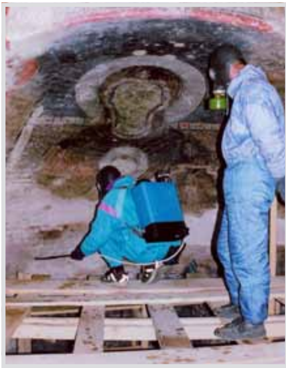
5. Timotesubani Church of the Virgin, conservation works on murals, treatment of biodeterioration with biocide.
