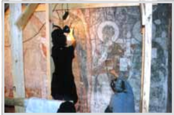
4. Timotesubani Church of the Virgin, conservation works on murals, consolidation of the paint layer
