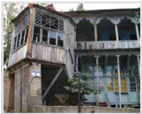
1. 3, Betlemi Street before restoration
