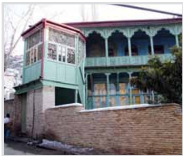
2. 3, Betlemi Street after restoration
