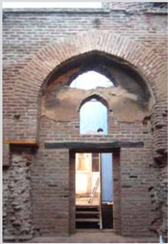
5. Ateshgah, interior after restoration
