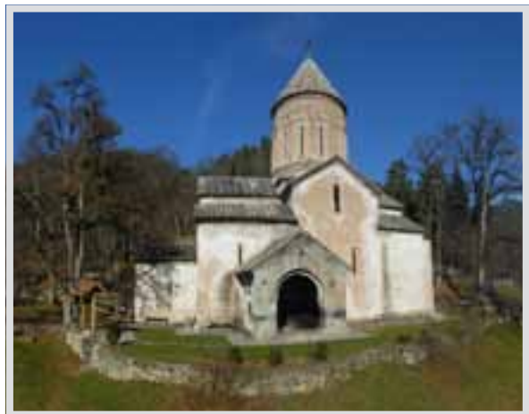
1. Timotesubani Church of the Virgin, exterior, view from the south
