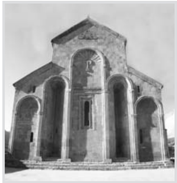
Reconstruction of Eastern façade
