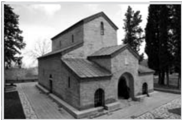
Bodbe, view from the north-west (9th century).
