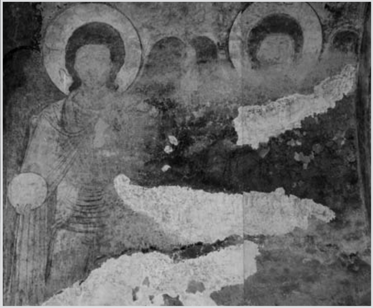
5. White fillings distracting from the reading of the original paint layer. Narthex, Kintsvisi.
