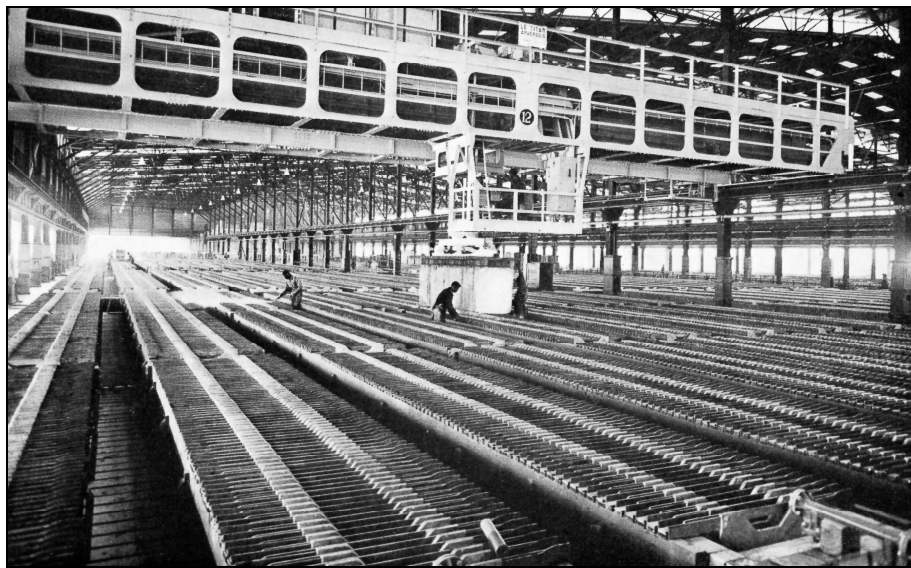
Figure 10. Zinc electrowinning plant.
