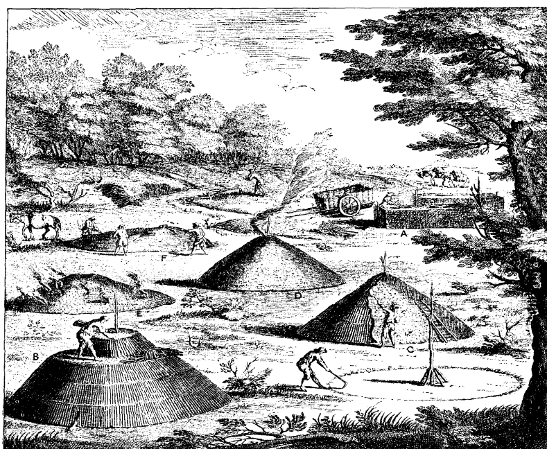
Figure 3. An early method for producing charcoal.
