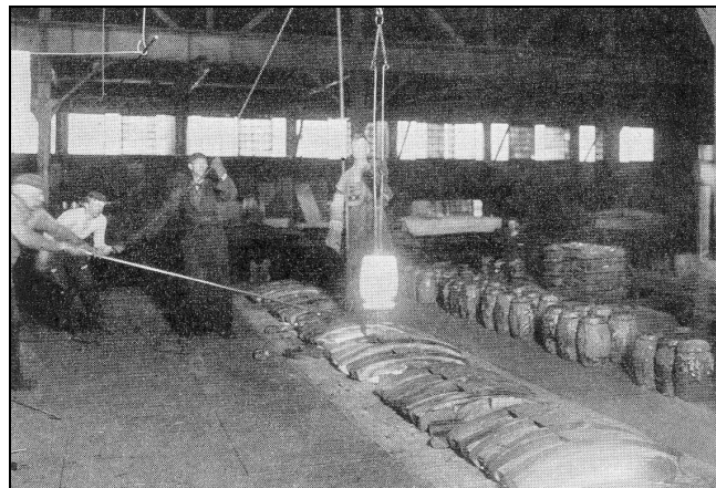
Figure 8. Production of cast steel: removing of crucible from cementation furnace.
