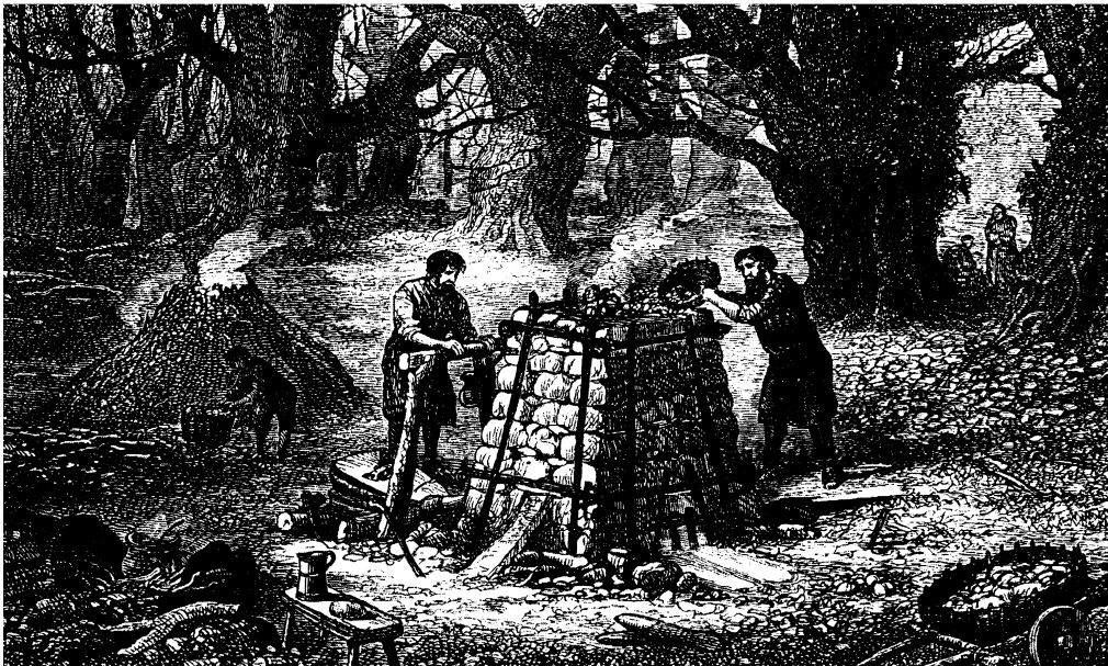
Figure 1. A typical furnace located in a forest for producing iron during the Roman Empire. The worker is operating bellows using his feet to blow air in the furnace. On the left hand is a kiln for producing charcoal from wood.
